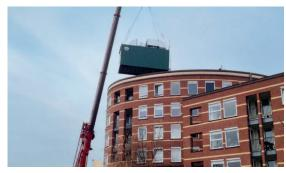
To achieve long term cost savings, the retirement home "Talma Borgh" decided to install a highly efficient CHP power plant. The project was realized in cooperation with with the dutch subcontractor "EKOB Energy BV". Because the tight spaces within the building made an integration into the basement impossible, an alternative location had to be found. In a spectacular process, the the CHP unit was lifted onto the roof of the 50 feet high building.
